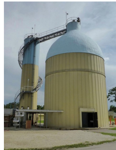
Figure 2: Example of an anaerobic digester.
